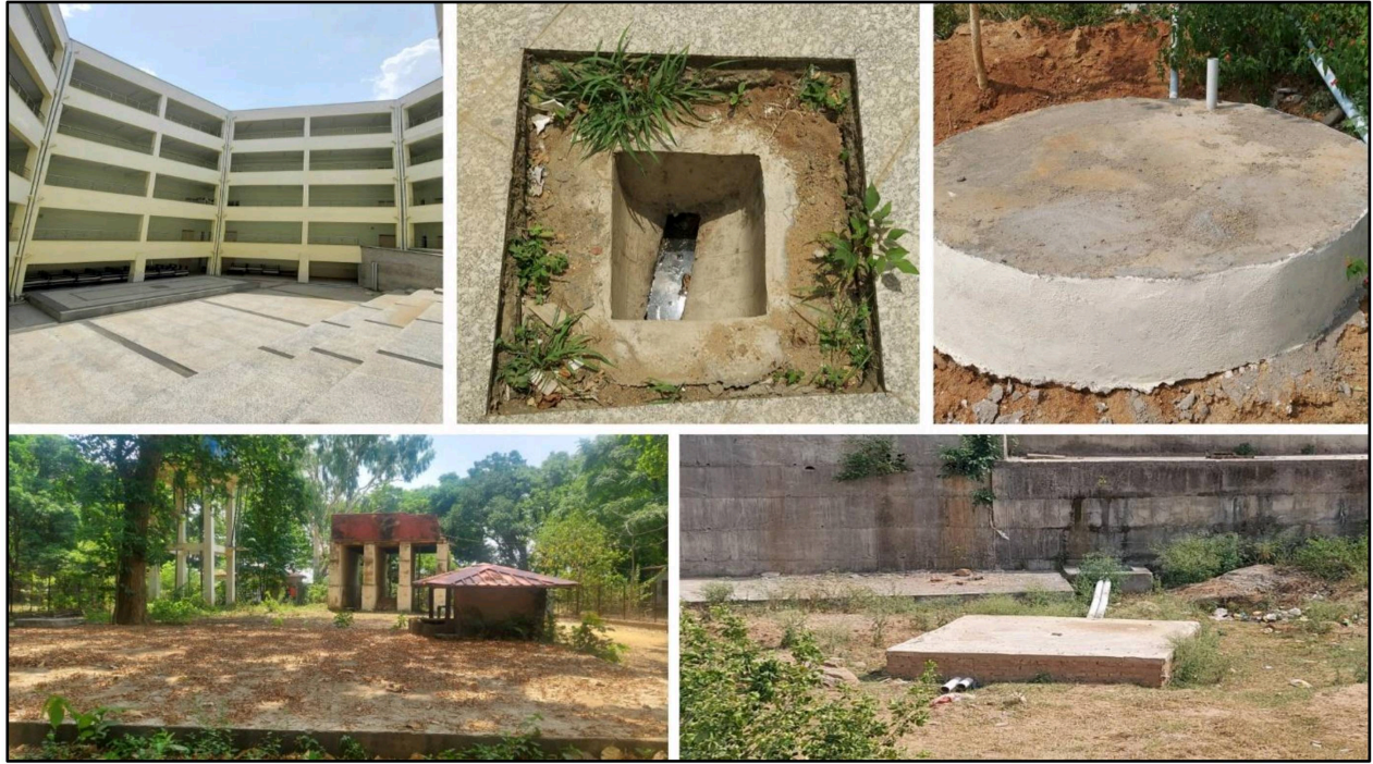
Figure 6. Rain water harvesting system and water recharging facilities in CUJ campus.
