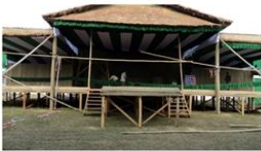
Cultural stage undergoing construction before the centenary celebration
